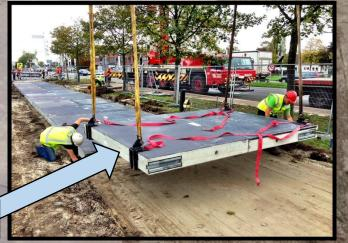
Solar cells imbedded in bikeway riding surface
